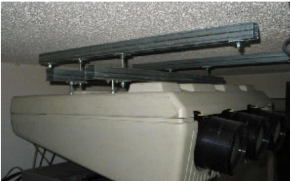
This is an Ampro 4000, which weighs in at 165lbs. Above the ceiling is attic space, so there are 2 more unistrut channels paired with the ones against the ceiling, the hidden struts sit across the top of 3 joists.
